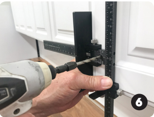
Position tool with stops as shown and drill hole through drill bushing
