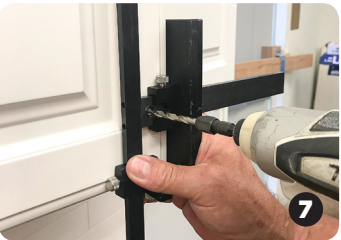
Reverse tool position onto opposite door and drill
