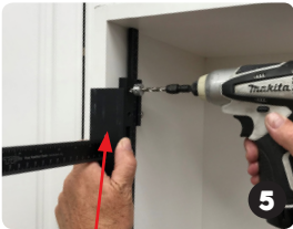
Set Large Stop to 37mm (industry standard). Drill top hinge plate holes
