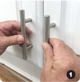
Place hardware (measure as needed) to find position you like; mark bottom hole location.
