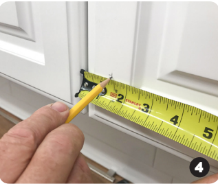
Measure from side of door to mark
