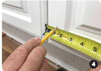
Measure from side of door to mark
