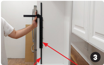
Slide Extended Ruler into Extension Bar , align any drill bushing with mark in cabinet, tighten thumb screws
