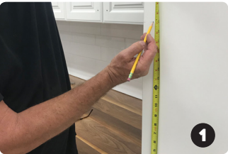
Measure and mark desired location of center hole to be drilled (we are drilling in sets of three)
