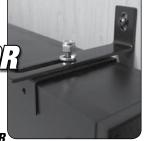
Secure the unit to the cabinet side wall. Pre-drill a pilot hole in the side wall before driving screw to prevent splitting the wood (use a 5/64 drill bit).
