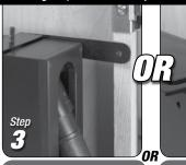
Secure the unit to the door frame. Pre-drill a pilot hole in the door frame before driving screw to prevent splitting the wood (use a 5/64 drill bit).
