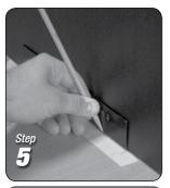
Positioning the Base Bracket Position the unit and make reference marks for the bracket. (A piece of masking tape to mark on works well.)
