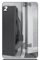
From the side, the unit should be positioned as far forward as possible while still allowing the cabinet door to close without hitting the hose handle.
