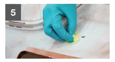
Prior to the application of 3M™ Instant Plastic Repair Patch, wipe area with supplied adhesion promoter and allow 5 minutes to dry.
