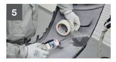
To achieve maximum strength apply 3M™ Crack Seal Tape and 3M™ Flexible Parts Repair Material to the back side of the repair area.
