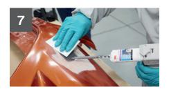
Using 3M<sup>™</sup> Applicator, apply 3M<sup>™</sup> Flexible Plastic Repair Materials to the damaged area. Spread and smooth and allow to dry for 20 minutes.
